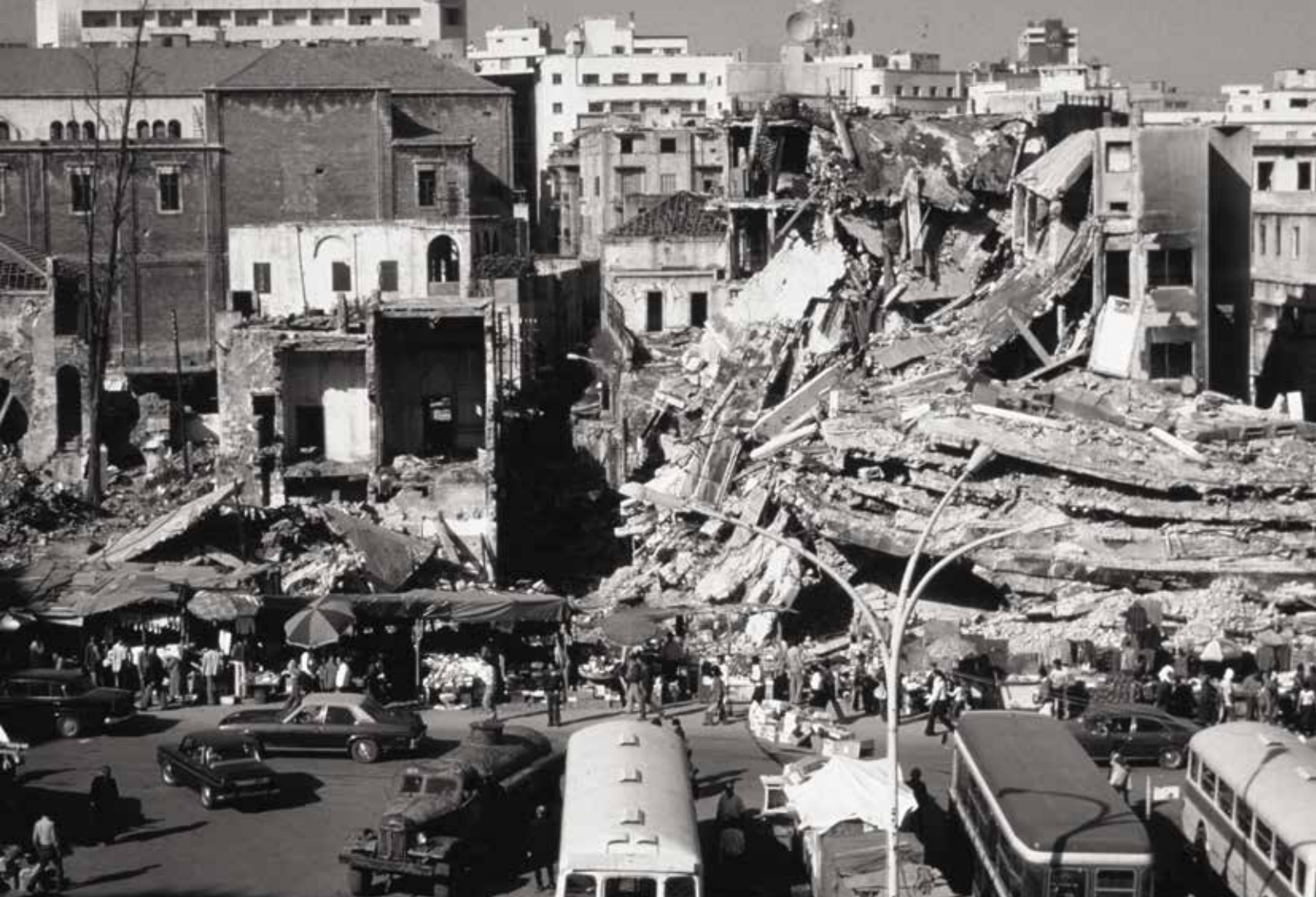
Place des Martyrs in Beirut showing gross damage during the civil war in Lebanon, 1975
